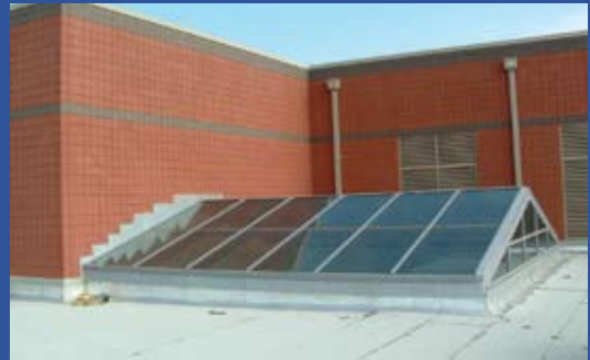
Architectural Block - After Nawkaw Application
