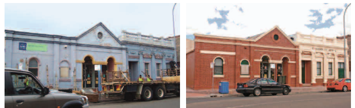
A Nawkaw Australian restoration and heritage project before and after staining.
